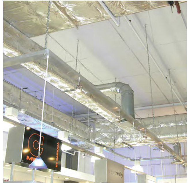
Exposed Under Soffit ceiling insulation below parking deck
